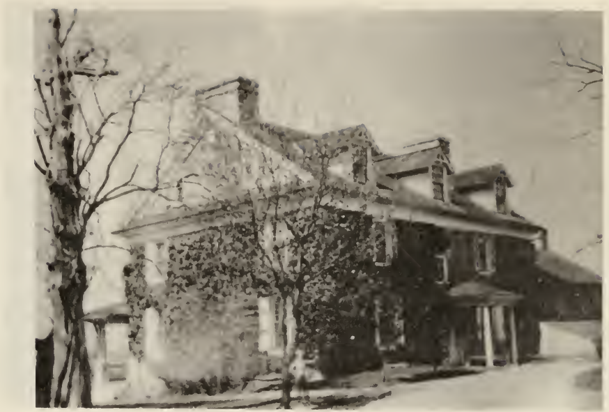
Figure 58. North elevation with three dropped-pendant style dormers, circa 1928. (Mutual Assurance Company, Policy No.10,478, June 21, 1928.)
